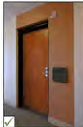
Example of proximity card reader system that is large in size with high tonal contrast compared to mounting surface for enhanced visibility.
