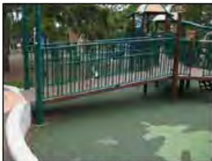
Ramp connected to elevated play components.
