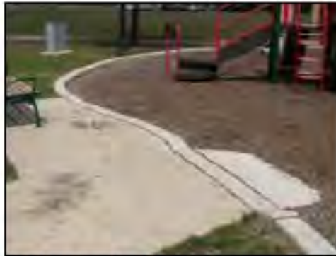
Curb ramp into play space where there is a level change between accessible route and play space.
